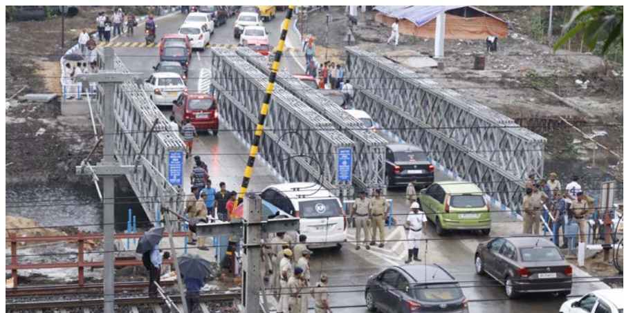
Portable Steel Bridge to Government of West Bengal
