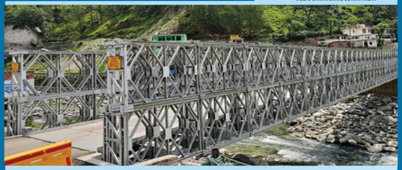
GRSE has developed new design Single Lane (4.25 M carriageway width) Modular Steel Bridge which is superior to the conventional Bailey bridge. GRSE is the sole indigenous manufacturer of Modular Steel Bridges (using 7 Feet Panel) in India and has been successful in supply and installation of ibid bridges in remote areas involving difficult terrains
