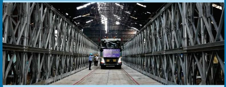
GRSE has embarked / endeavoured in the field of designing and manufacturing Portable Modular Steel Bridges that have the distinct advantages over conventional Bailey Bridges in terms of Load Carrying Capacity, Maximum Single Span and Cost benefit (by way of reducing weight). The design of such Modular Steel bridges has been successfully vetted and validated by SERC-CSIR, Chennai. The ibid bridges cater to both IRC as well as AASHTO Load Classes.
